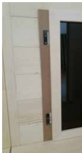
Fig. 53: Installing the backrests of the bench
