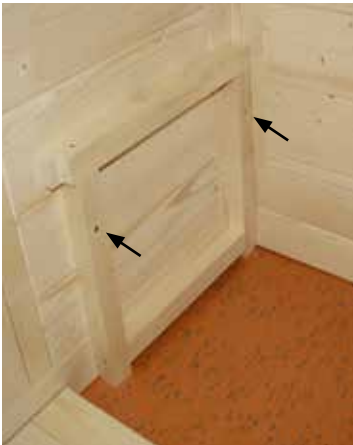
Fig. 32: Installation of the bench cushion
