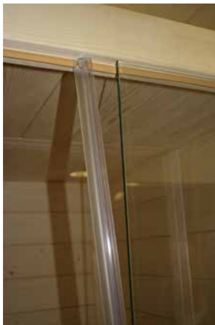
Fig. 20: Installing the door insulation strips
