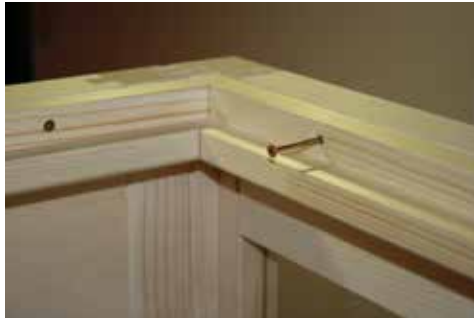
Fig. 15: Roof support slats installation
