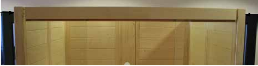
Fig. 14: Attaching the skirting
