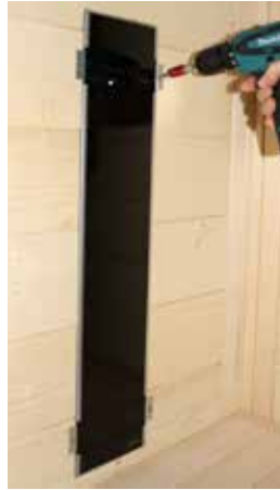
Fig. 41: Install the rear radiator (infrared radiator ECO 350)
