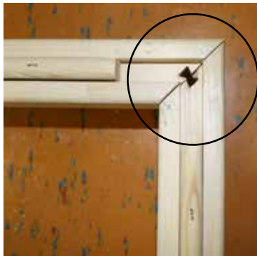
Fig. 2: Connect the floor frame elements
