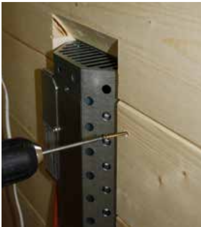
Fig. 42: Installing the read radiator blind
