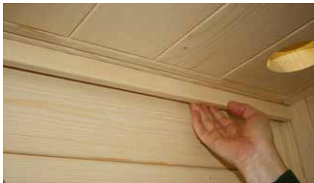
Fig. 38: Glueing the LED strips in place
