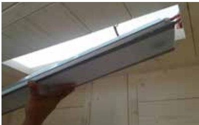
Fig. 50: Installing the colour light
