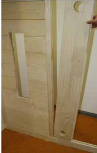
Fig. 6: Install the electrical element in place
