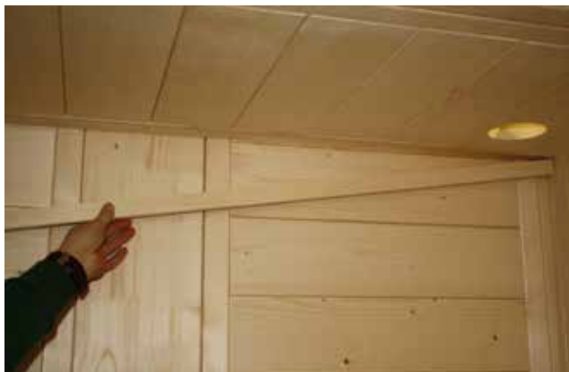
Fig. 37: Installation of the LED cover strip
