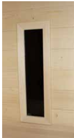
Fig. 42: Installing the read radiator blind
