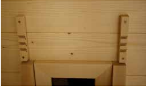
Fig. 54: Installation of the headrests
