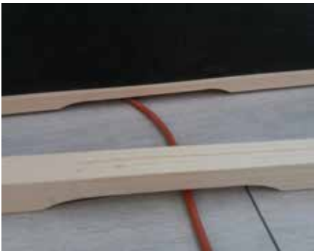
Fig. 35: Inserting the stiffener bar for the Vitamy IR thermal plates.
