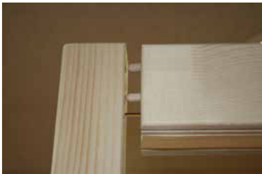
Fig. 13: Installing the skirting over the glass front
