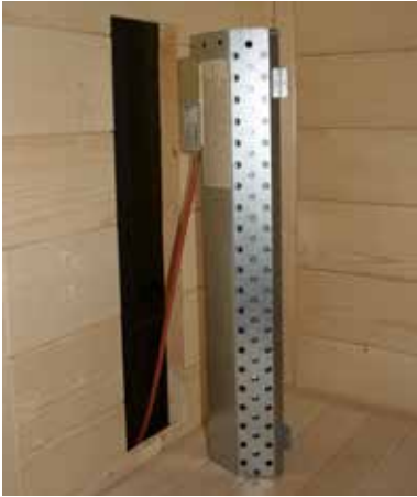
Fig. 41: Install the rear radiator (infrared radiator ECO 350)
